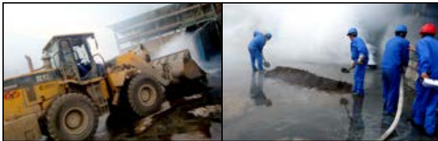
●装载机运来磷矿粉堵修围堰
